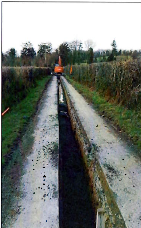
Plate 1: Typical Trench Construction within roads Ducts
